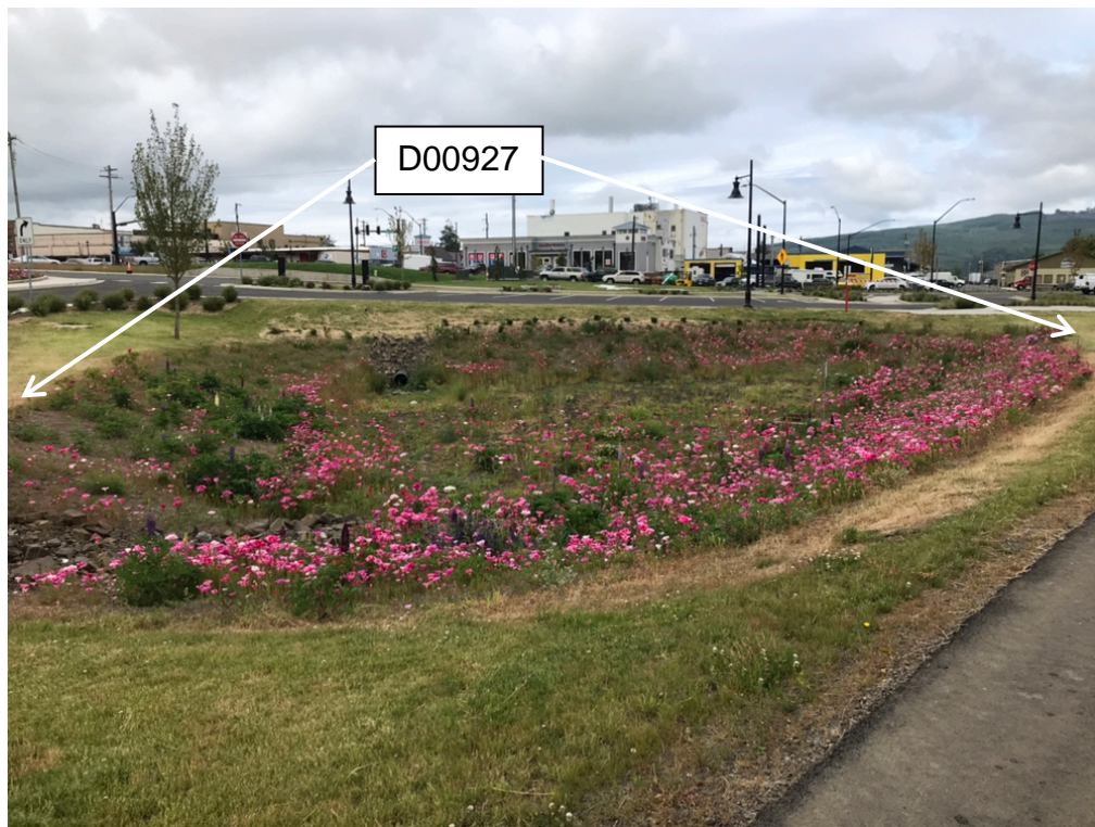
Figure 1: DFI No. D00927, looking West
