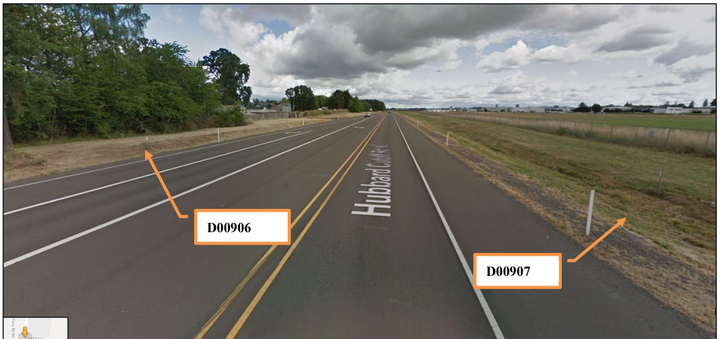
Figure 1: DFI No. D00906 and D00907 looking north along highway
