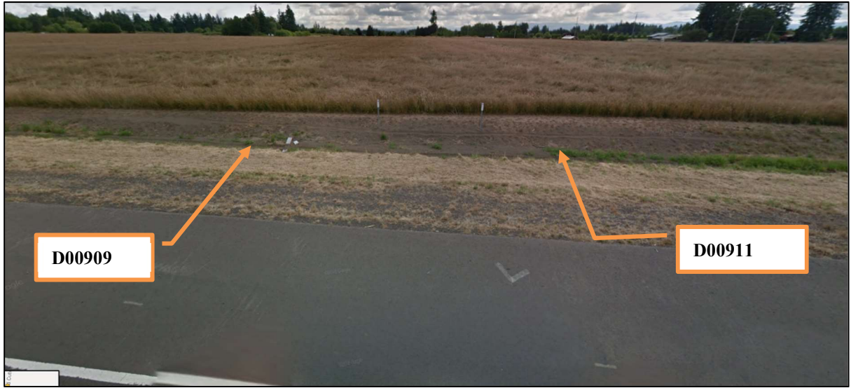
Figure 2: DFI No. D00909 and D00911 looking east from highway shoulder
