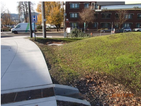
Figure 7: Looking west. Auxiliary inlet near center, marked 'C' on operational plan and profile.
