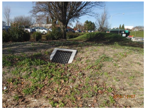
Figure 8: Looking north. Inlet marked 'D' on operational plan and profile.
