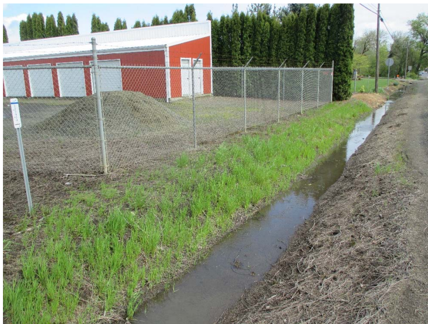
April 2017 - Facility Location following Construction
