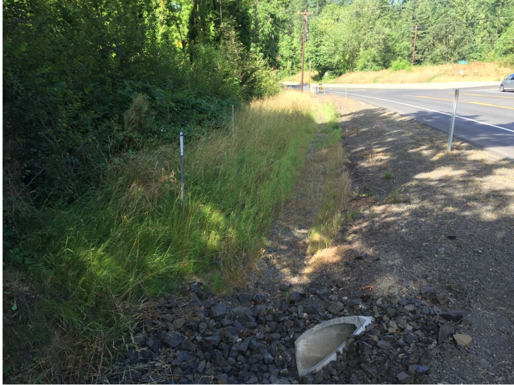
Photo 3: Looking west at one of the two double culverts, bioswale outlet
