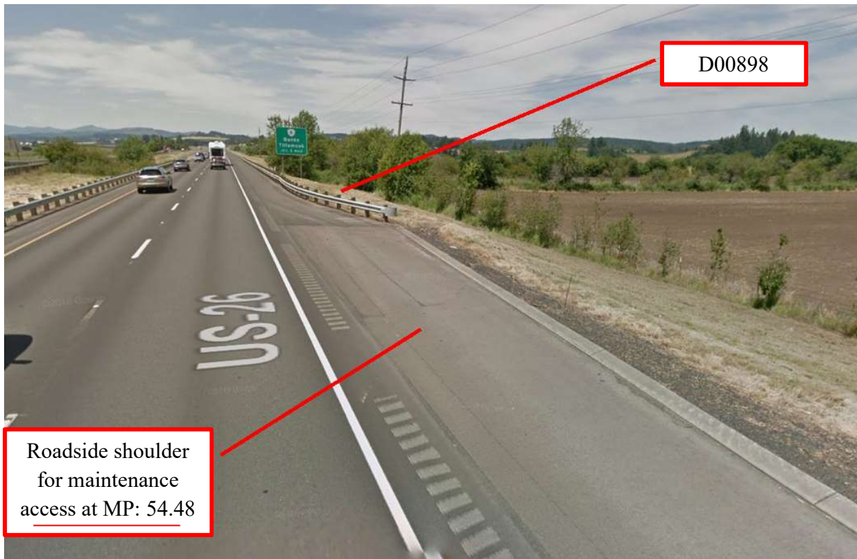
Figure 4: Maintenance access for D00898 for westbound traffic
