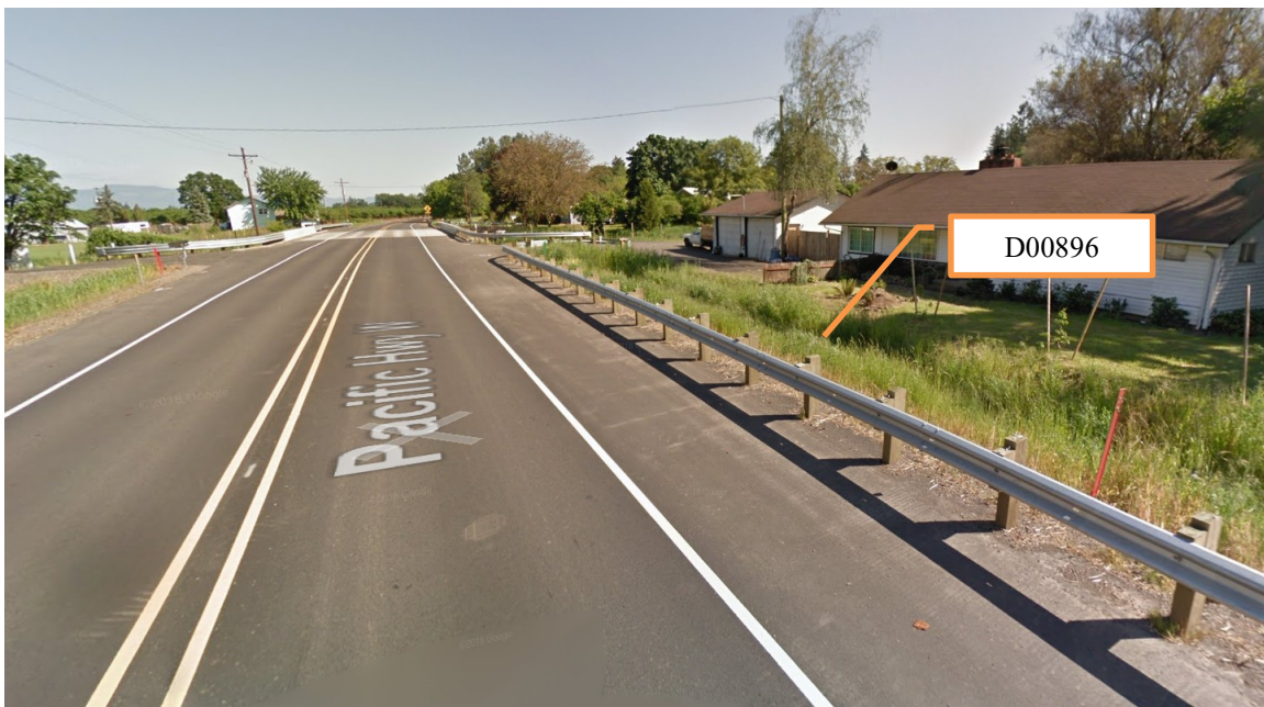
Figure 1: Looking south at the bioswale located along west side of Pacific Highway West (99W)
