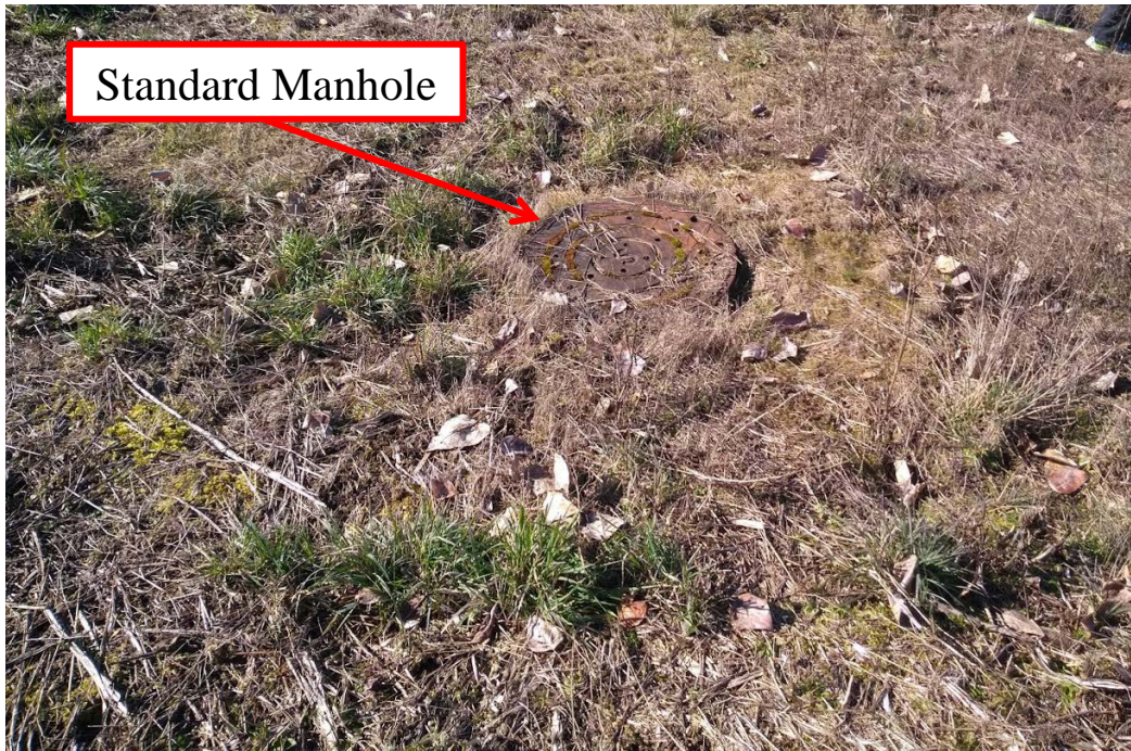
Figure 5: Water flows through standard manhole, then through swale
