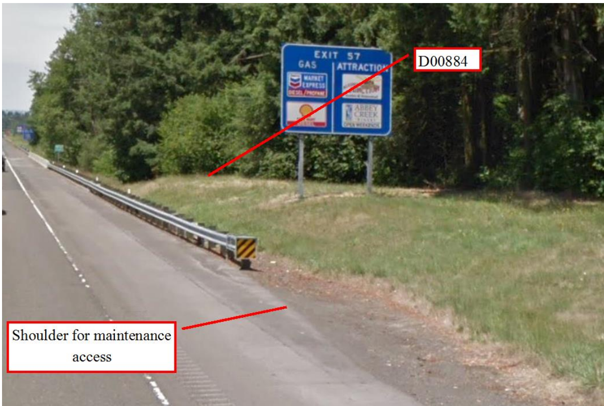
Figure 4: Maintenance access for D00884 for westbound traffic
