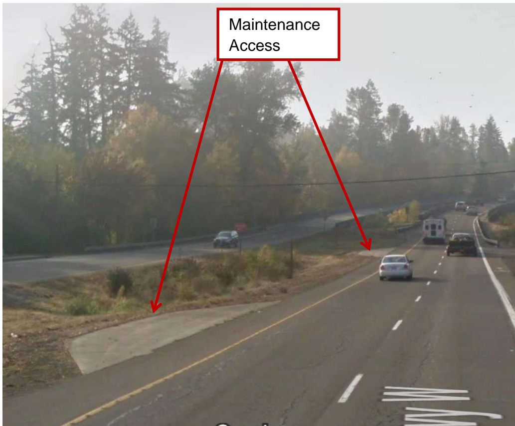
Figure 3c: D00876, looking south toward Tualatin River Bridge, 2 SB maintenance pads
