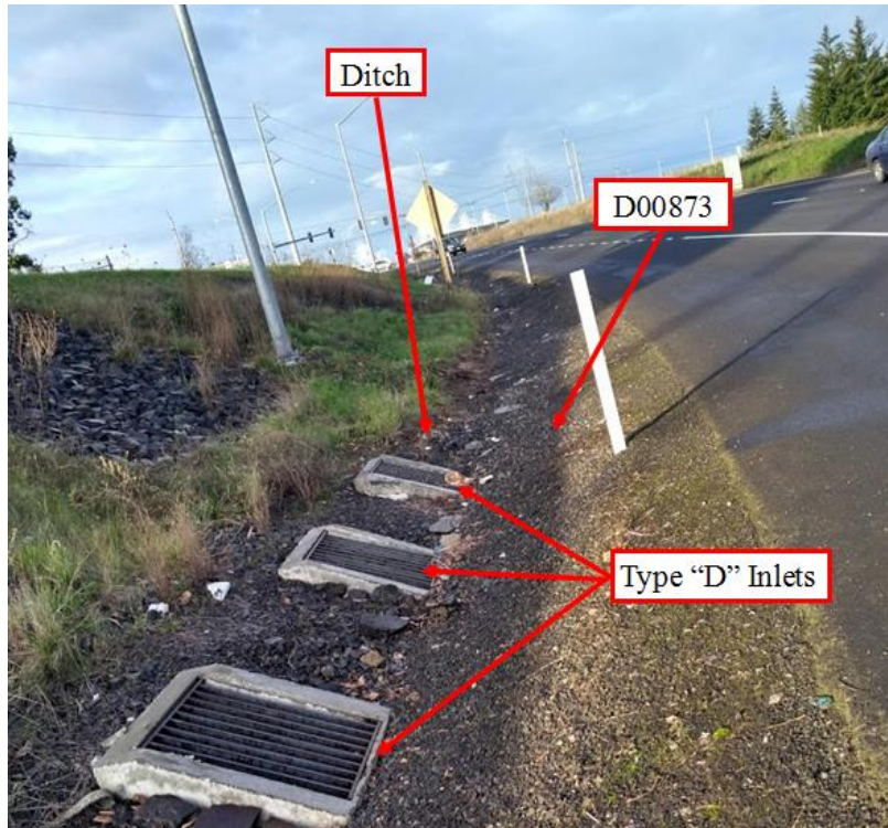
Figure 6: Components of D00873
