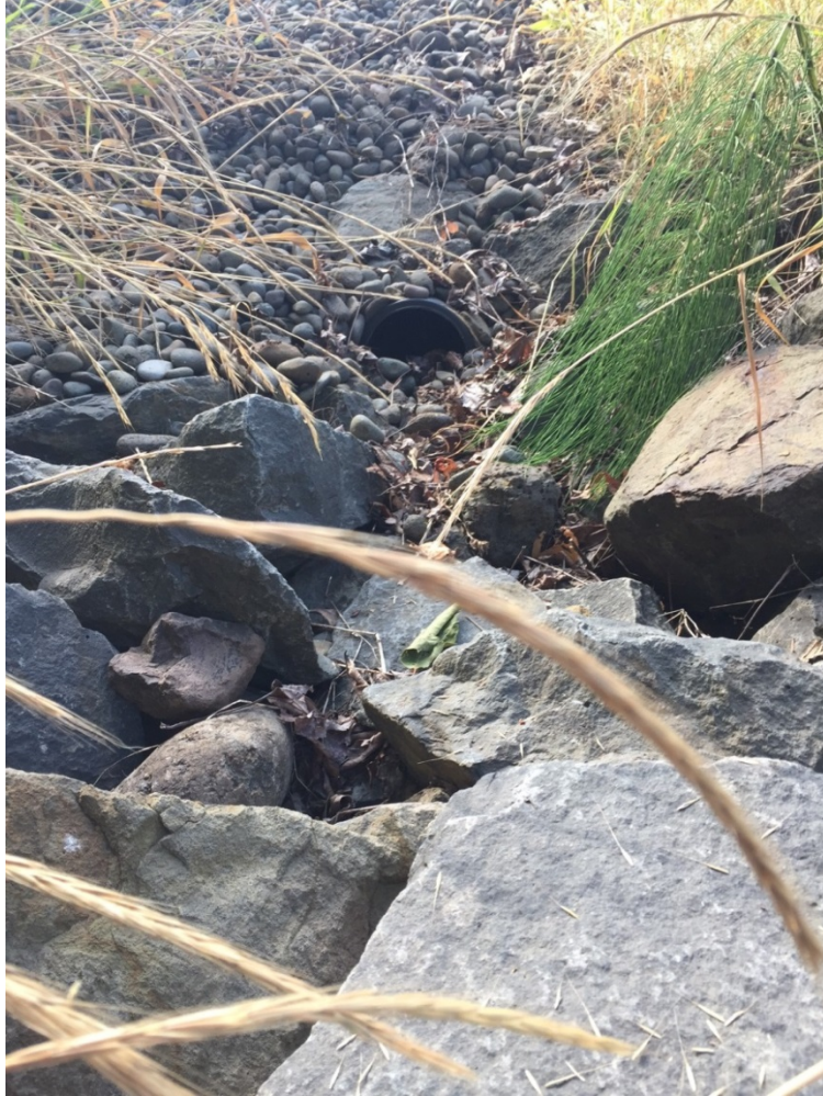
Photo 3: Outfall drain into riprap basin, looking east towards bioslope.
