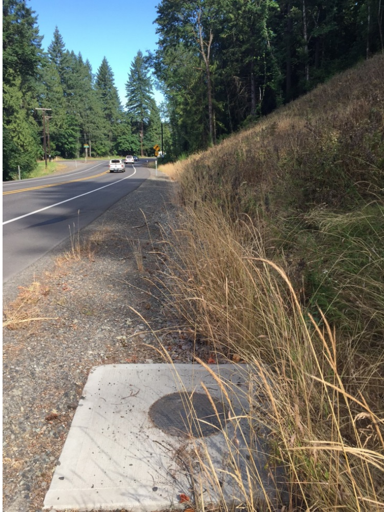
Photo 2: Looking west at the top of the iron cover and concrete casing of one of three PVC inlets along the bioslope.
