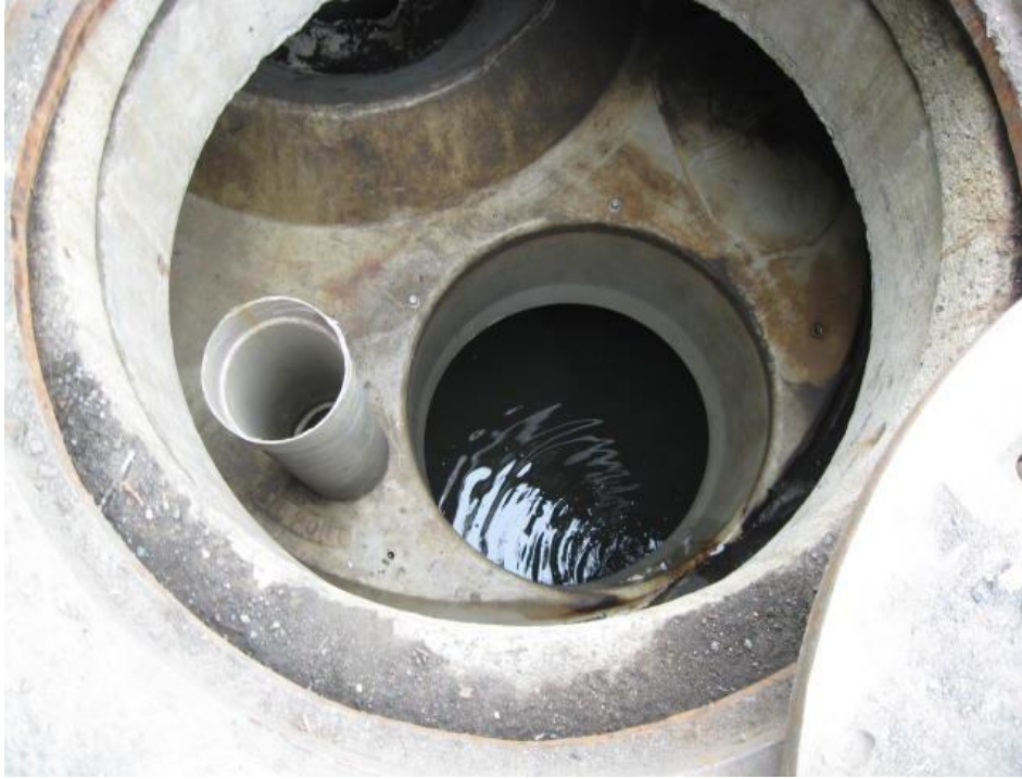
Photo 2: Interior view of Stormceptor water quality manhole.
