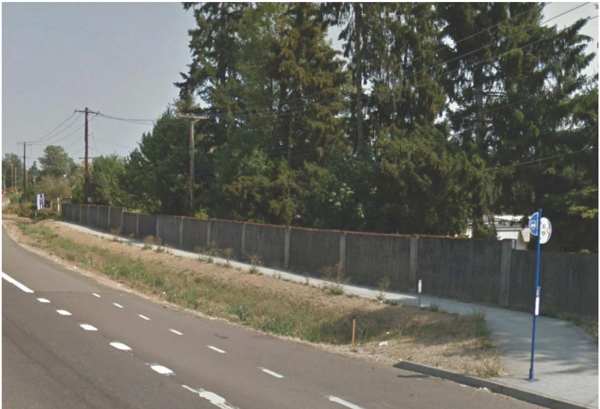
Figure 1: DFI No. D00851, looking east
