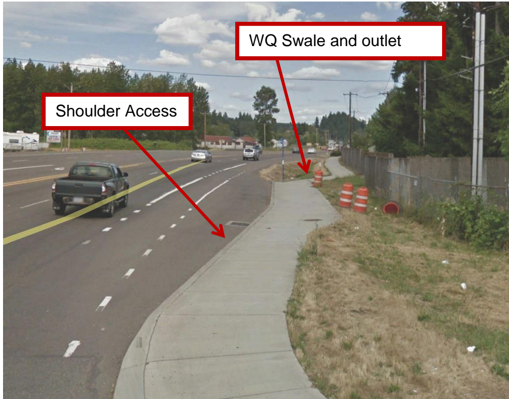
Figure 3: Maintenance Access for Eastbound traffic]
