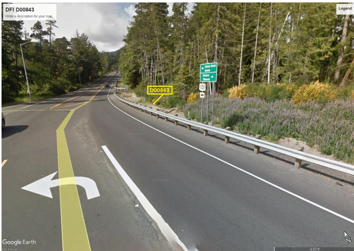
Figure 1: DFI No. D00843, looking North
