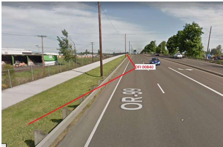
Figure 1: DFI No. D00840, looking north
