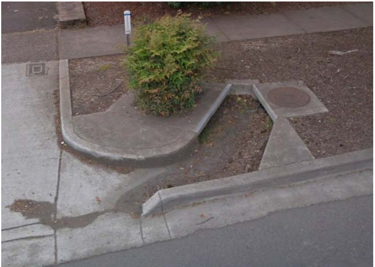
Figure 1: DFI No. D00831, looking west
