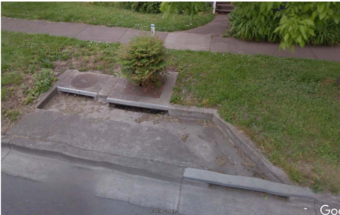
Figure 1: DFI No. D00828, looking west
