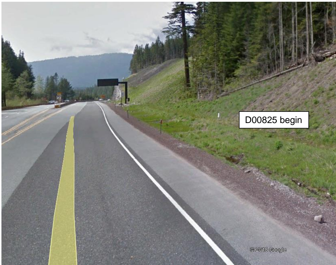
Figure 1: DFI No. D00825, looking west
