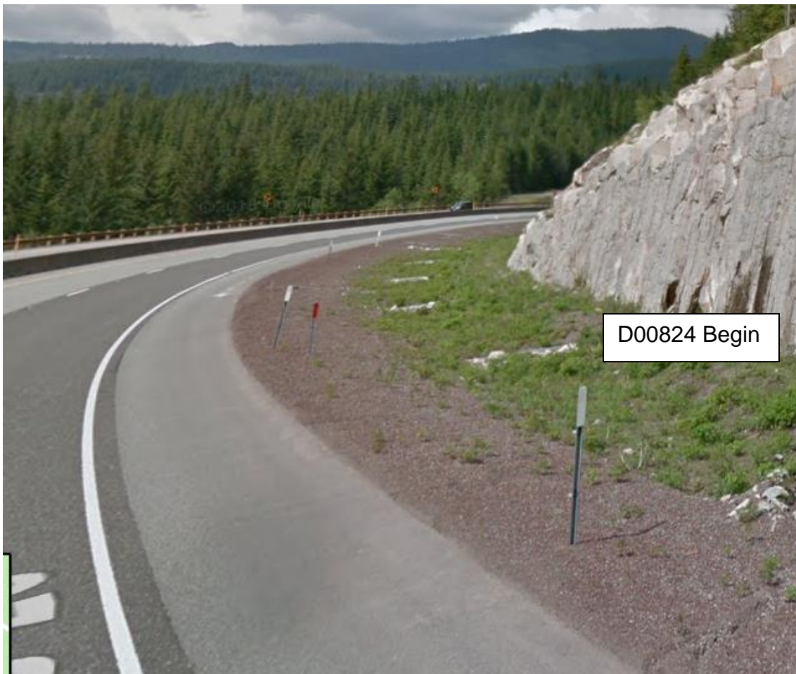
Figure 1: DFI No. D00824, looking west
