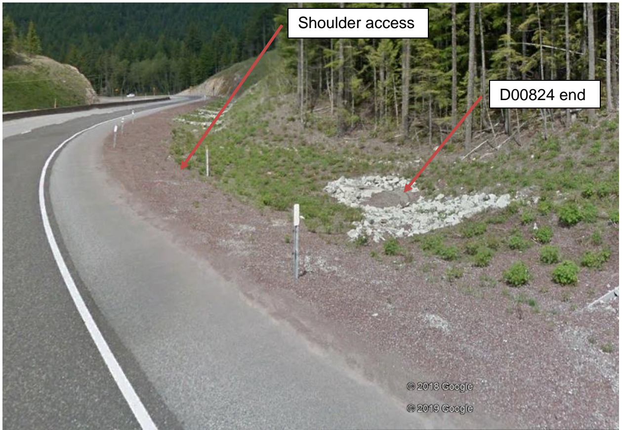
Figure 3: Eight foot shoulder access, facing west
