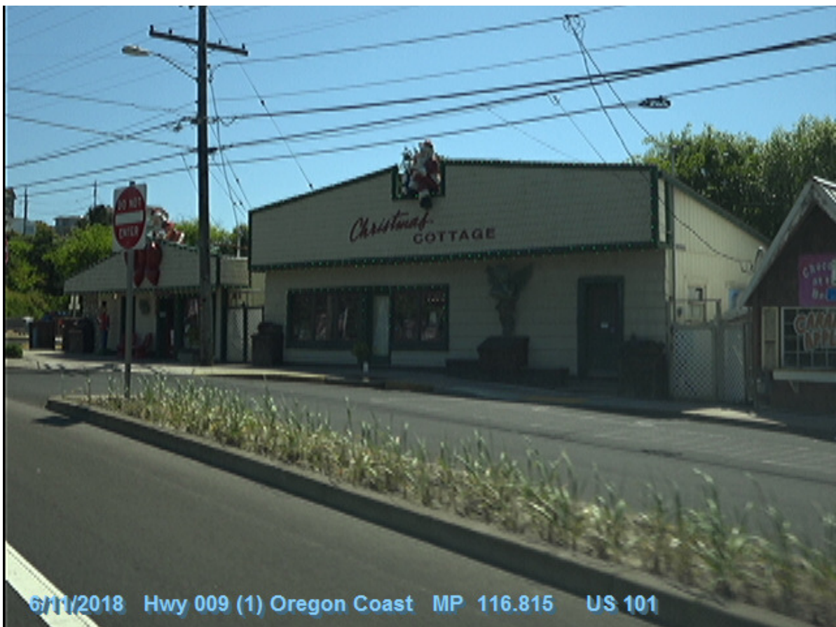
Figure 1: DFI No. D00822, looking North
