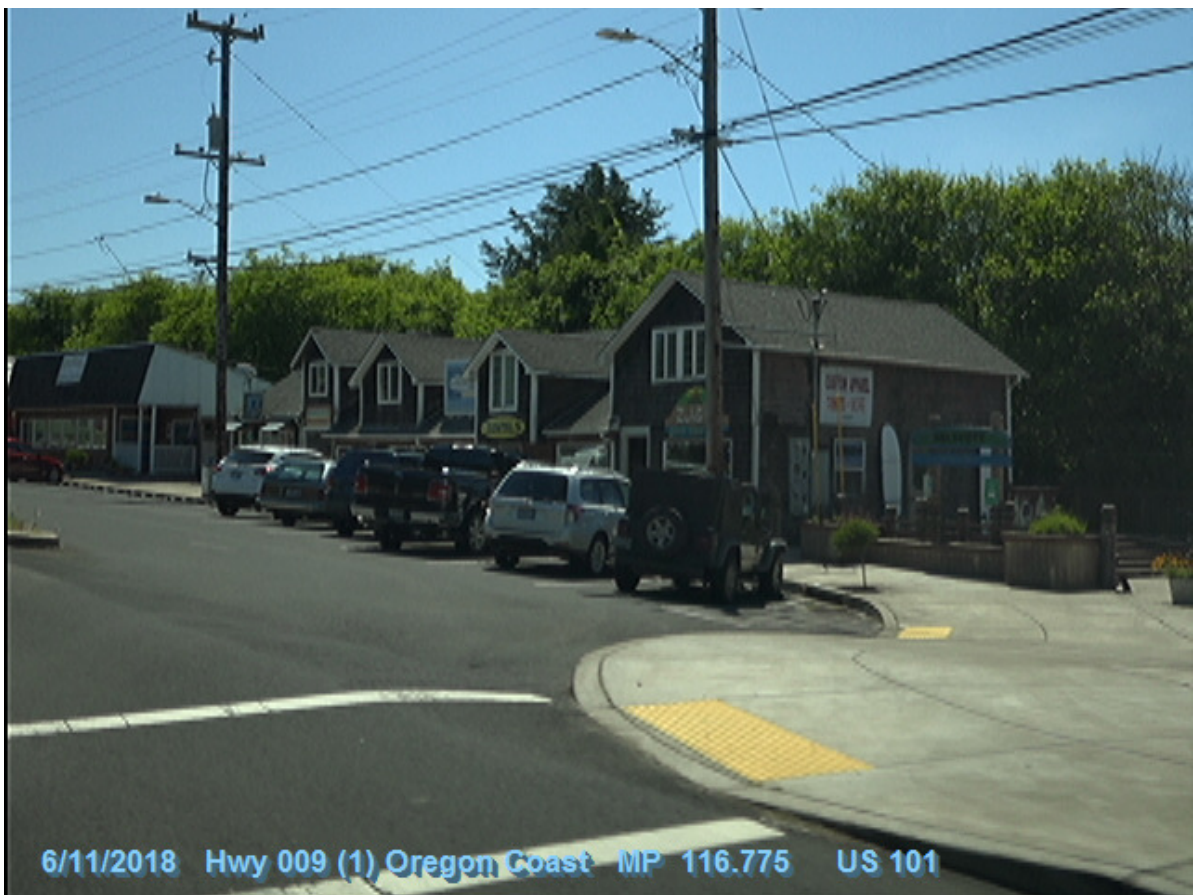
Figure 1: DFI No. D00820, looking North
