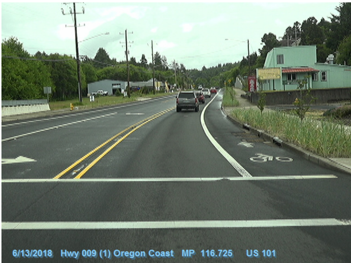
Figure 1: DFI No. D00819, looking North
