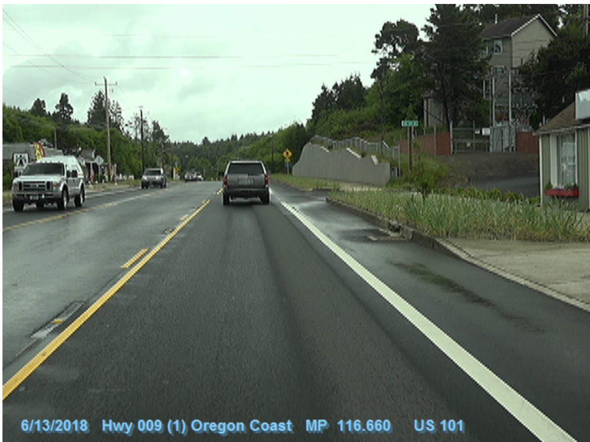
Figure 1: DFI No. D00815, looking North
