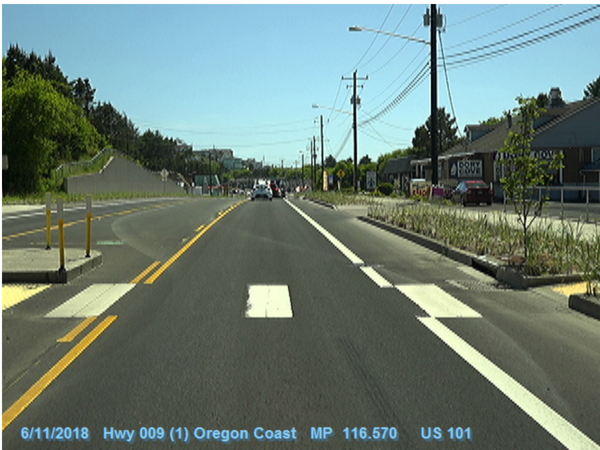
Figure 1: DFI No. D00810, looking South
