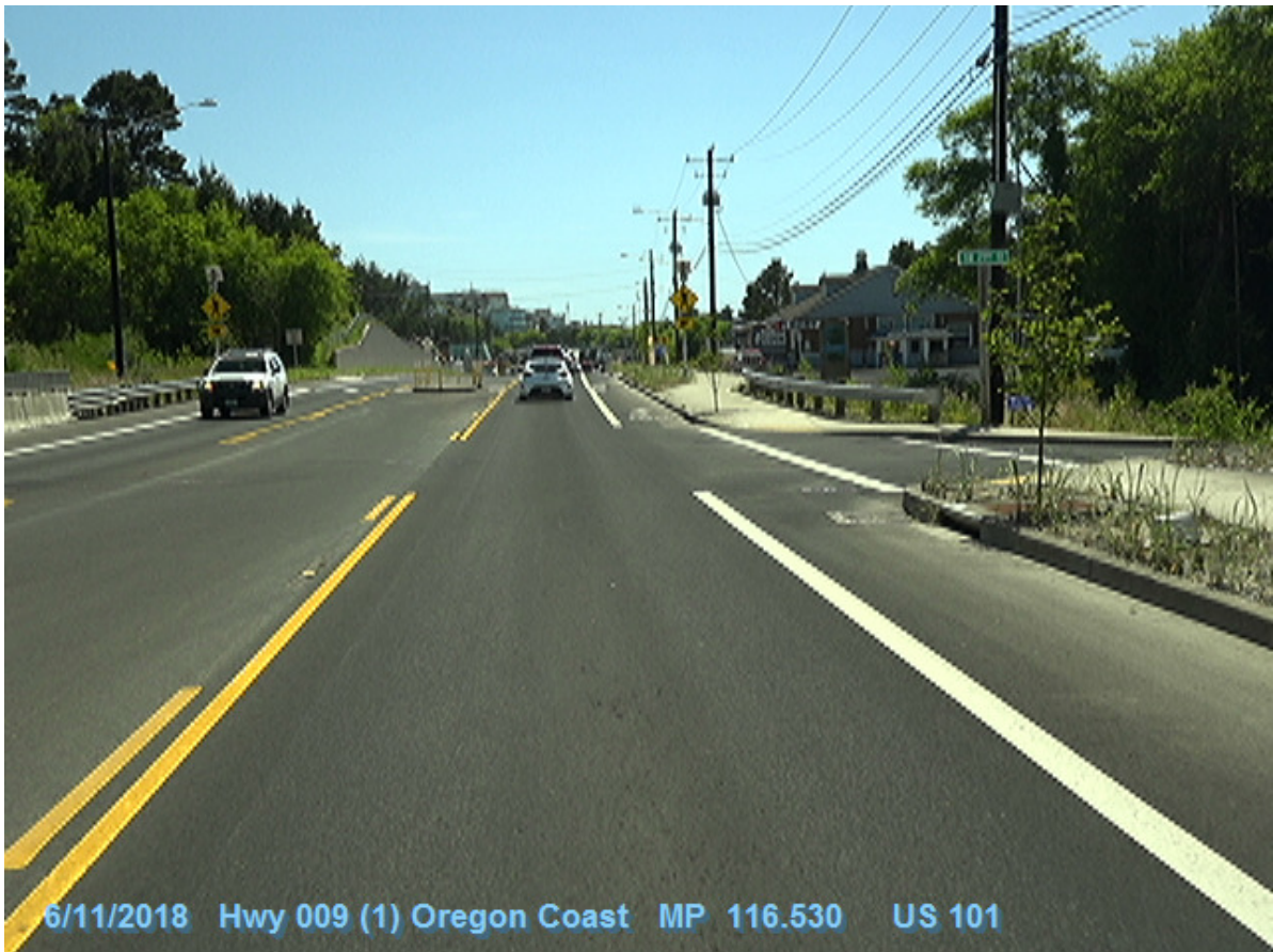
Figure 1: DFI No. D00807, looking South
