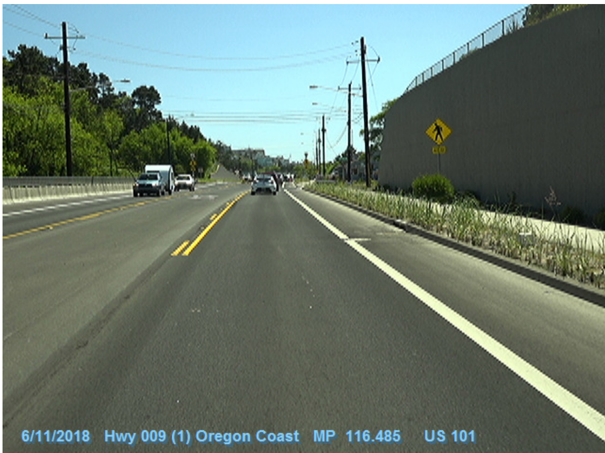
Figure 1: DFI No. D00806, looking South
