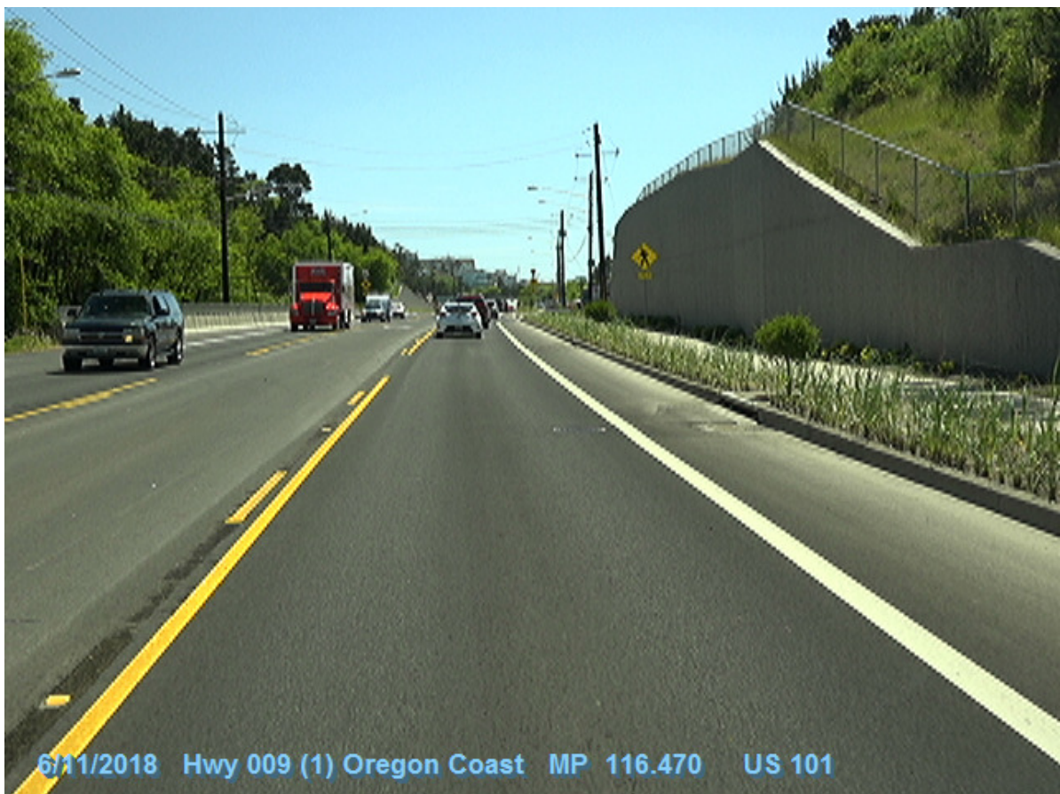
Figure 1: DFI No. D00805, looking South
