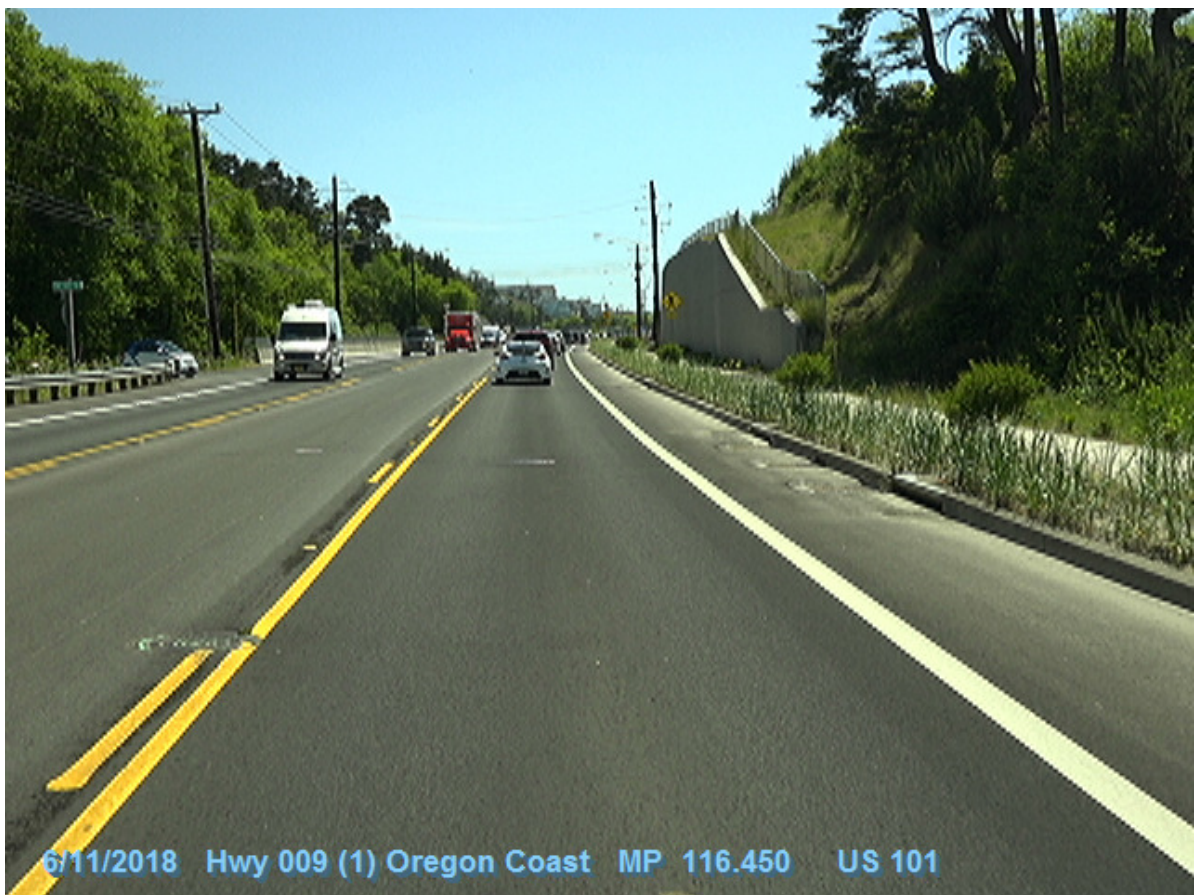
Figure 1: DFI No. D00803, looking South
