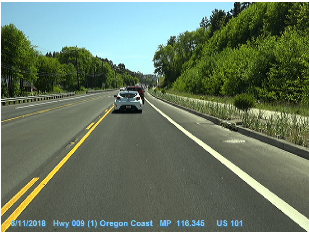
Figure 1: DFI No. D00798, looking South
