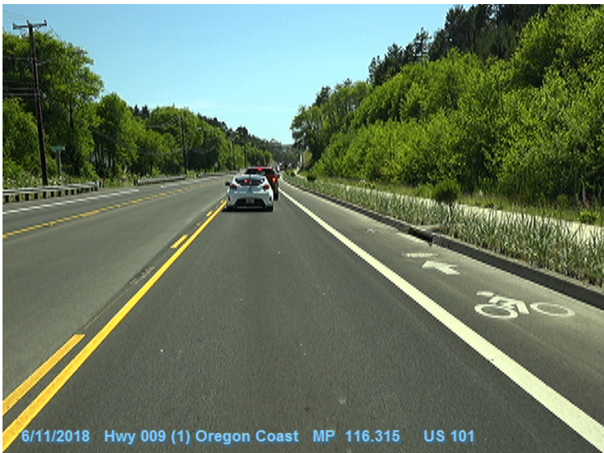
Figure 1: DFI No. D00797, looking South
