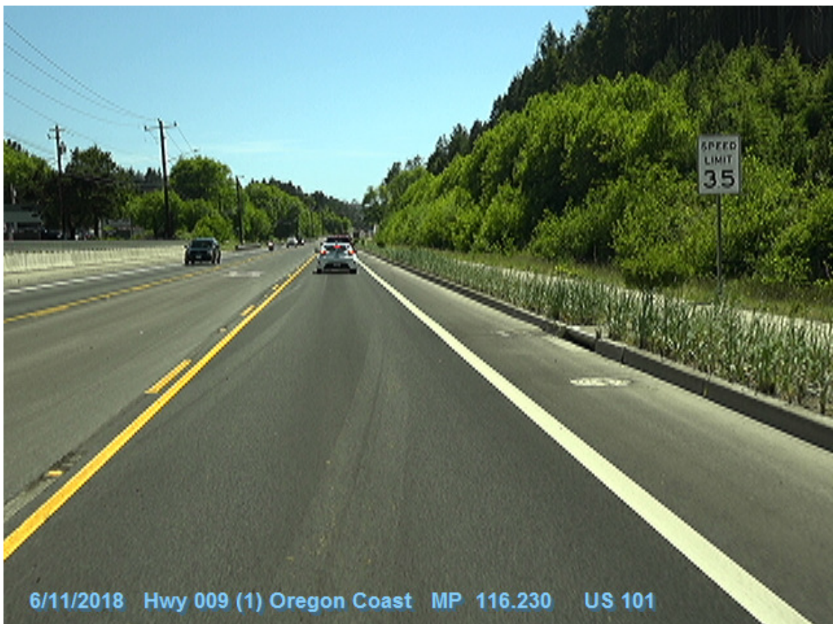
Figure 1: DFI No. D00795, looking South
