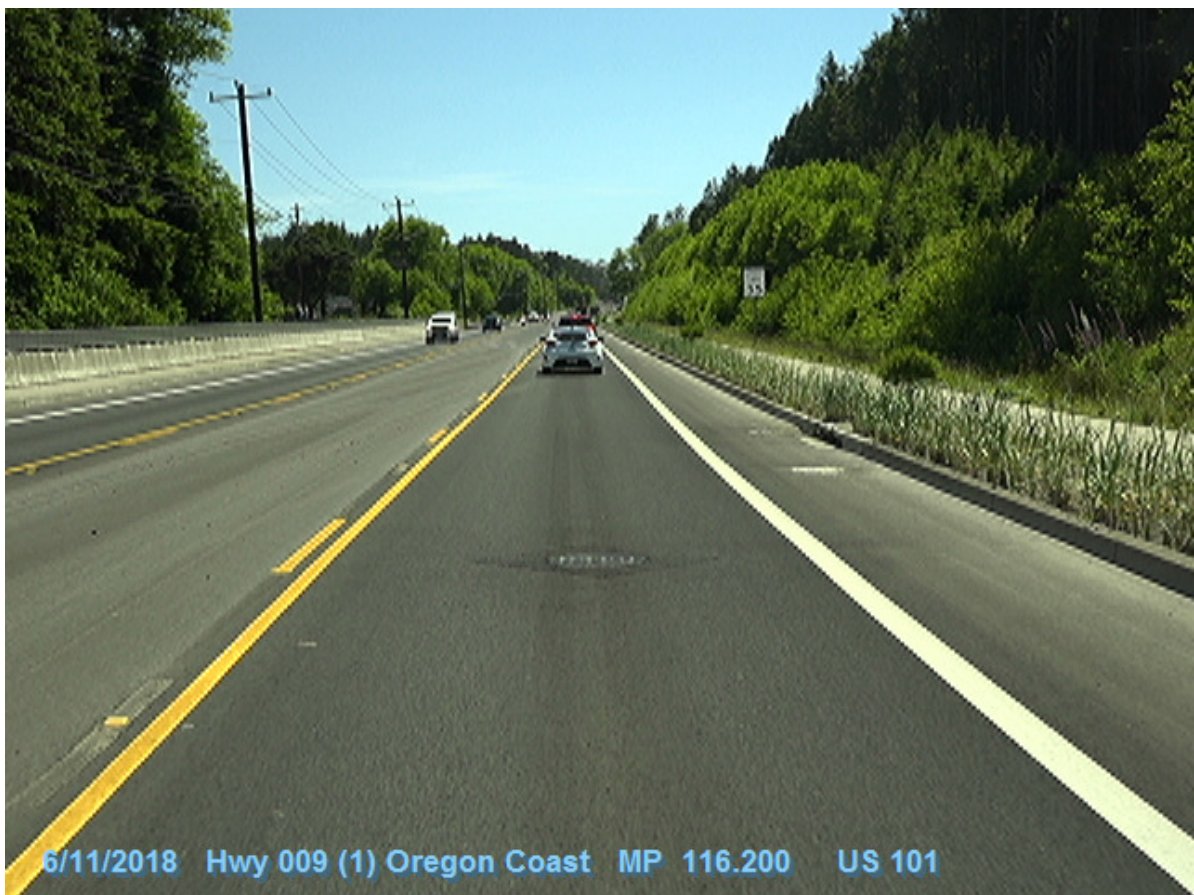
Figure 1: DFI No. D00793, looking South
