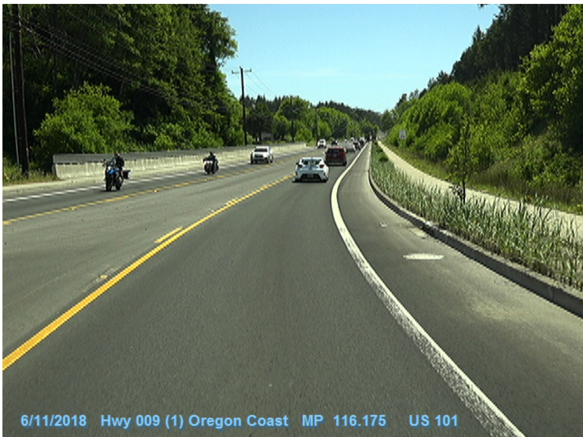
Figure 1: DFI No. D00792, looking South
