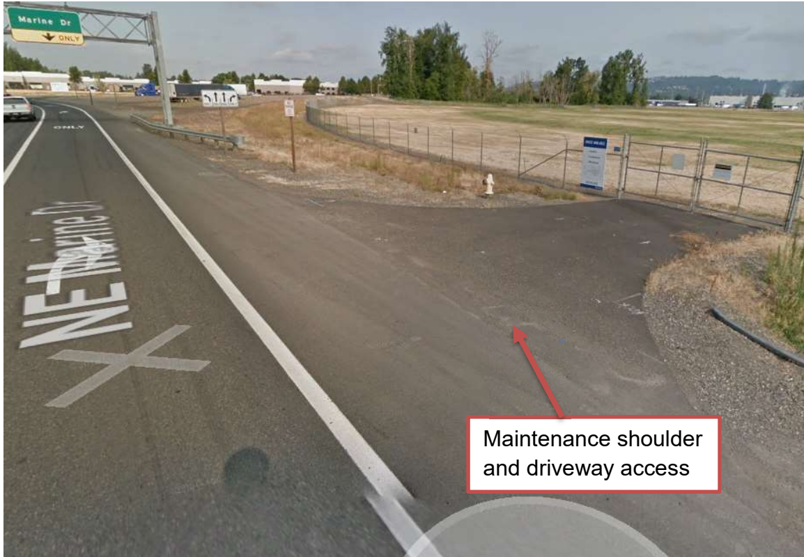
Figure 3: Looking west at Infiltration Slope
