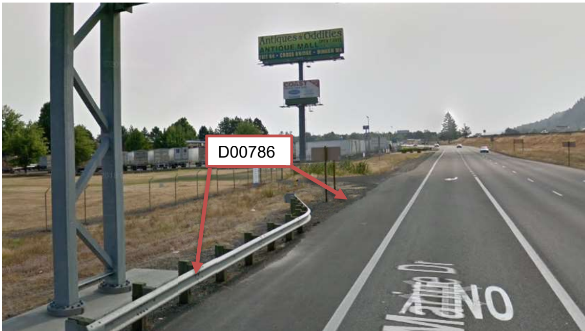
Figure 1: DFI No. D00786, Looking East
