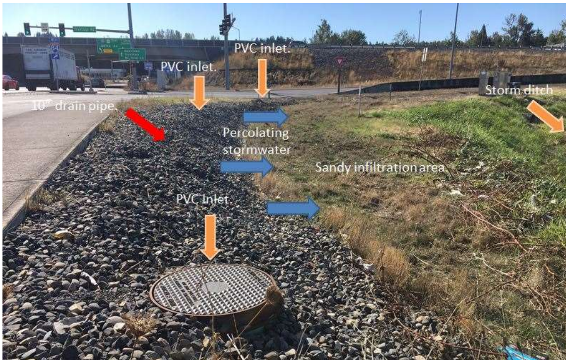
Figure 5: Looking south at facility (Marine Dr. on the left)
