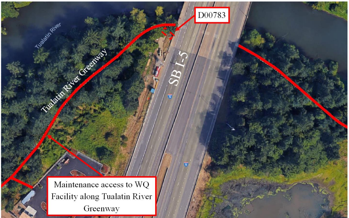
Figure 6: Maintenance access to WQ Facility
