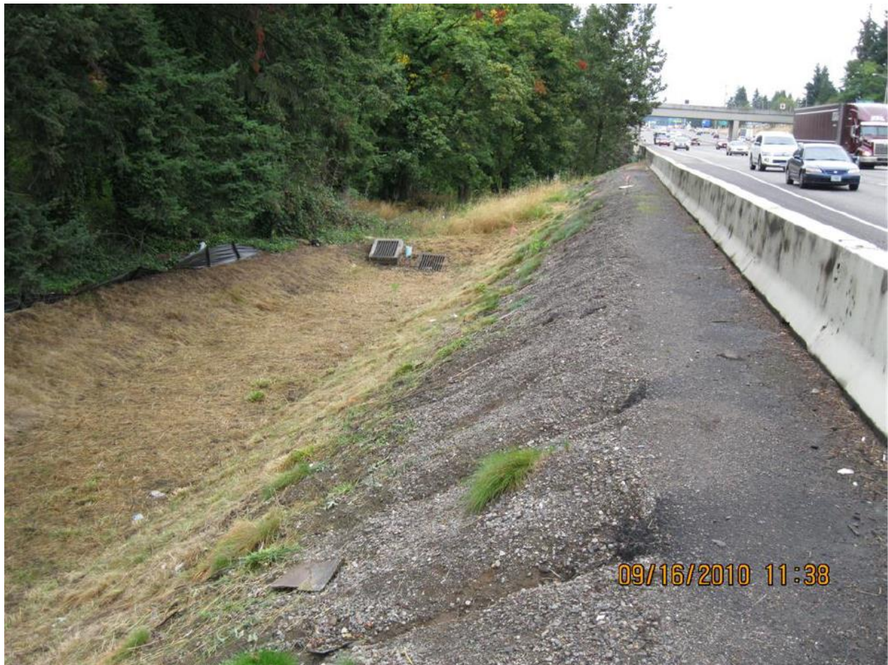
Figure 1: DFI No. D00782, looking southwest
