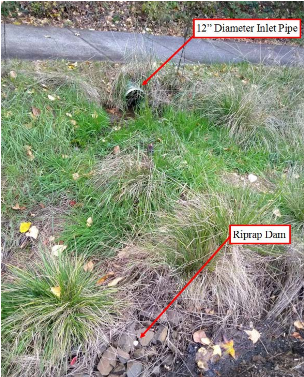
Figure 5: Piped Inlet in middle of swale
