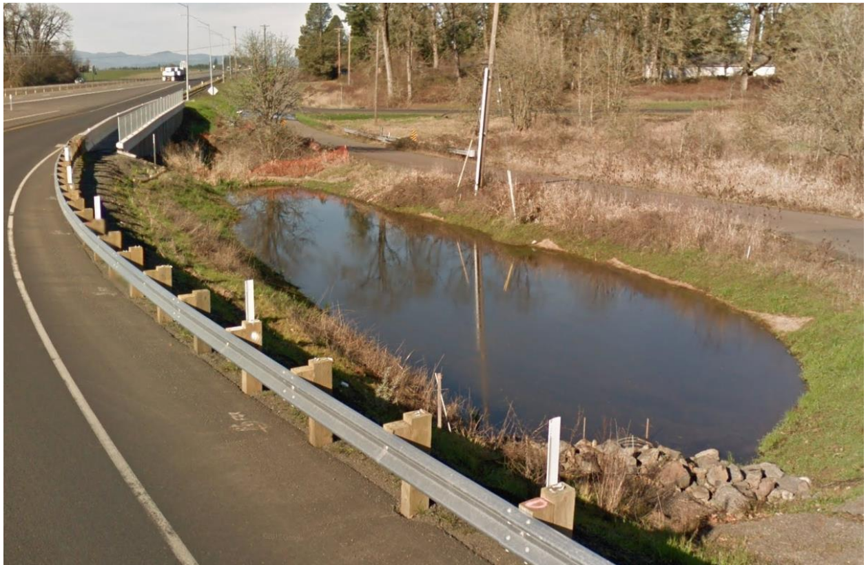
Figure 1: DFI No. D00773, looking northwest (photo taken Feb 2016)
