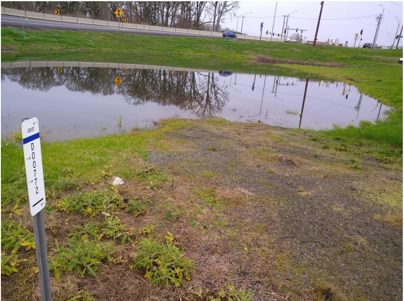
Figure 1: DFI No. D00772, looking
