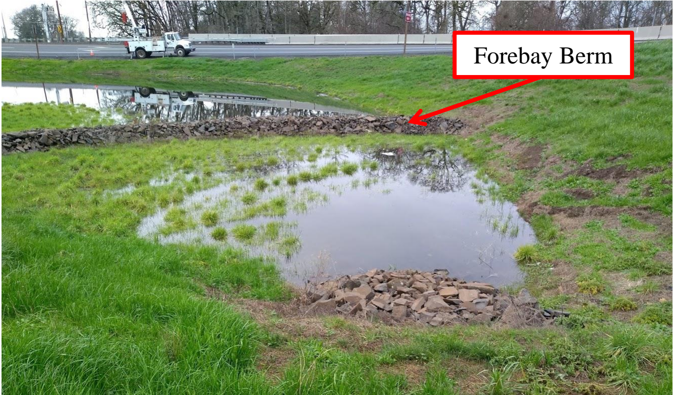
Figure 5: Components of detention pond
