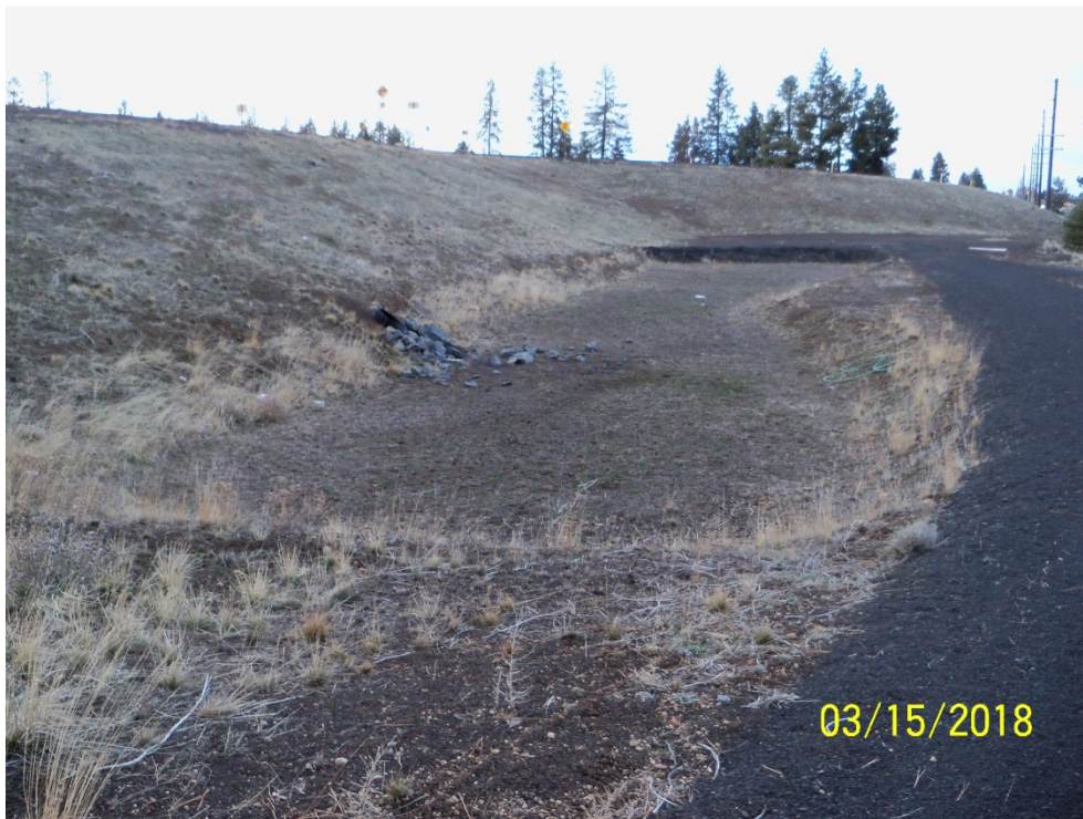
Figure 1: DFI No. D00746, looking North
