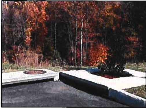
1. Inspection of Filterra and surrounding area
