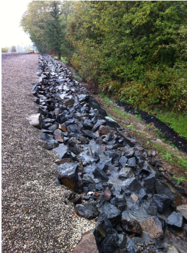
Figure 8: Looking north at riprap channel
