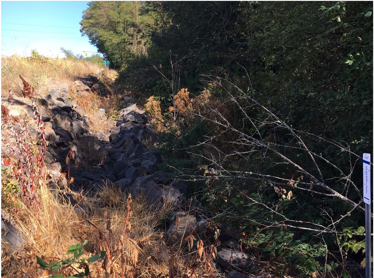
Figure 1: DFI No. D00727, looking north
