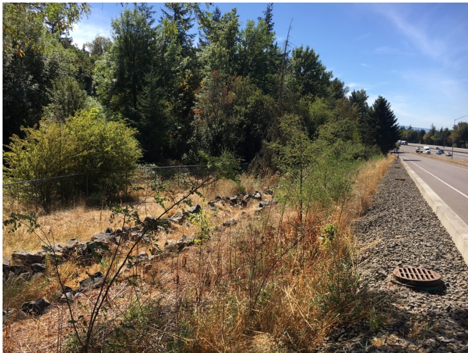
Figure 13: Looking southeast at bioslope facility with inlet #1 visible
