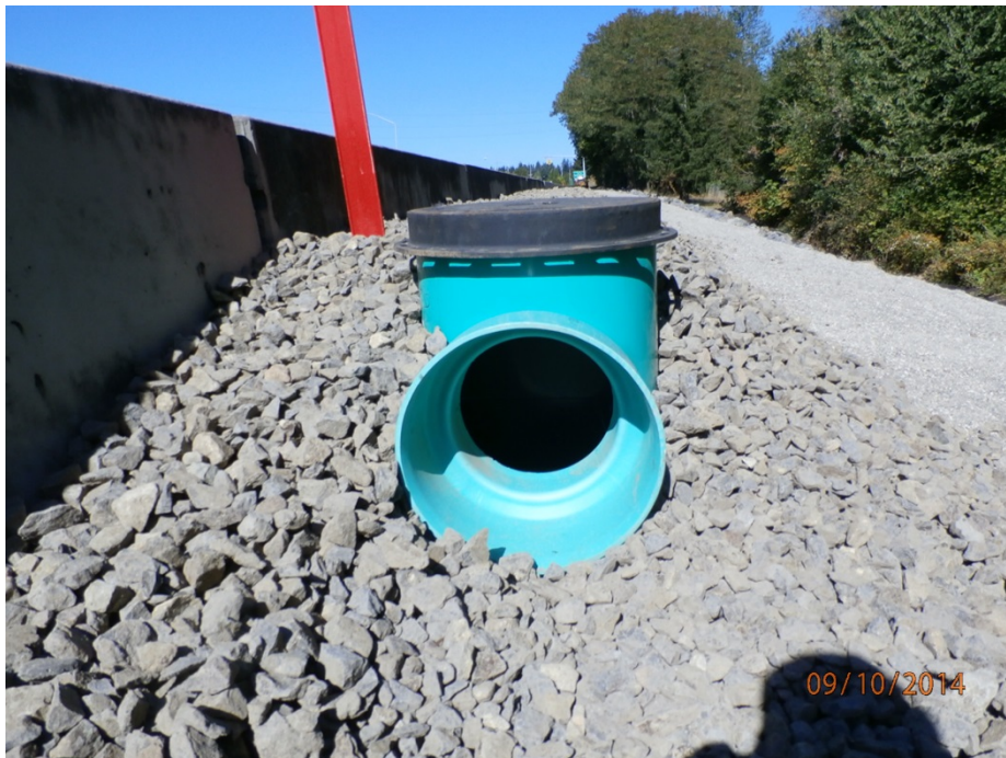
Figure 9: Looking north at inlet #6. Overflow outlet visible
