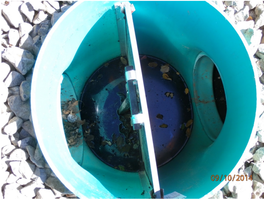
Figure 11: Aerial view of PBV inlet (1 of 6) with weir
