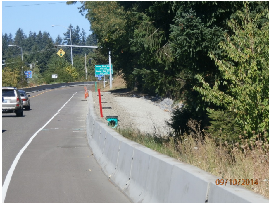
Figure 6: I-5 Northbound off ramp exit 294, looking north.
