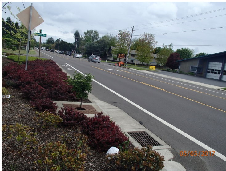
Figure 1: DFI No. D00724, looking East
