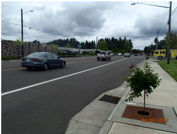
Figure 1: DFI No. D00721, looking East
