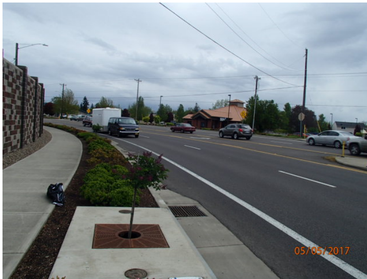
Figure 1: DFI No. D00716, looking East
