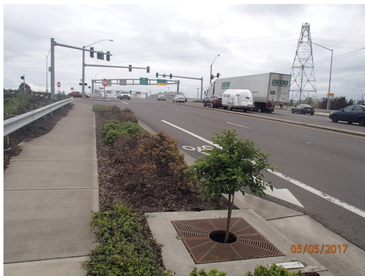
Figure 1: DFI No. D00715, looking East
