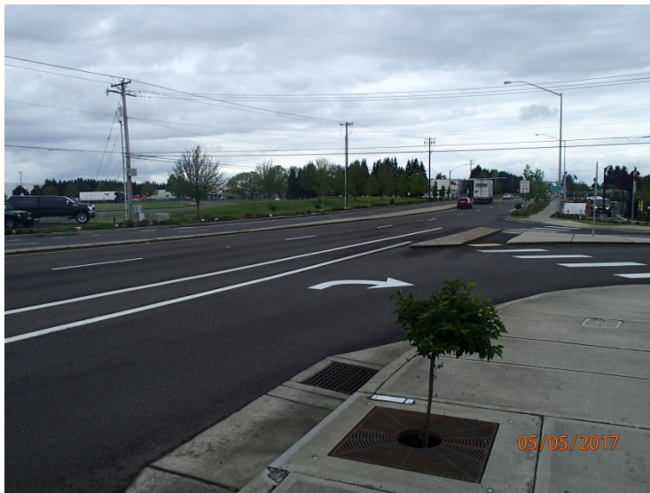
Figure 1: DFI No. D00712, looking West
