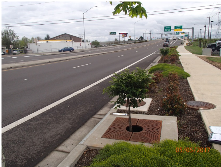
Figure 1: DFI No. D00710, looking East
